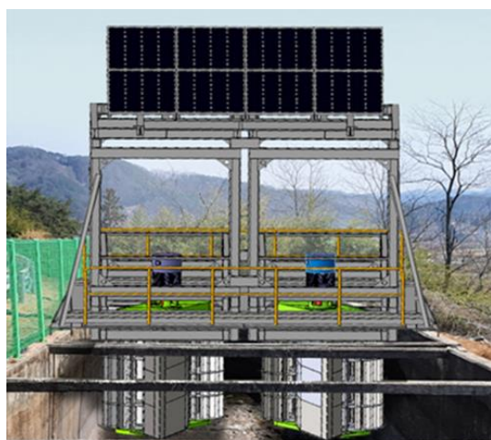
Figure 1. A hybrid combination of solar and small hydropower plants.
