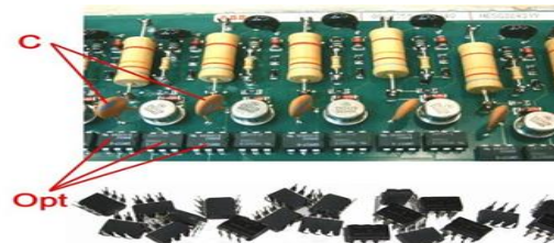
Fig. 2. A part of DPR logic input module of REL316 type with damaged capacitors C and failed opto couplers Opt.
