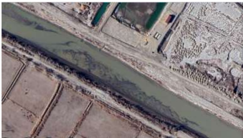
Fig. 3. Siltation and erosion in the Anasai main canal in the Republic of Karakalpakstan (2022)
