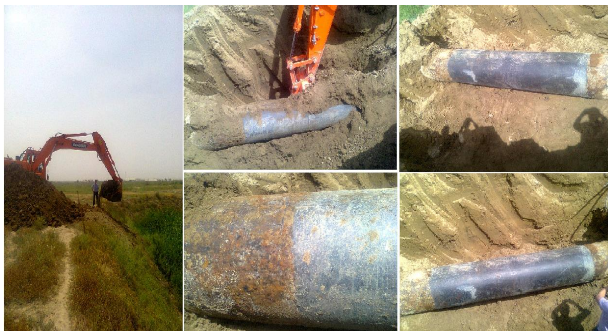
Figure-1. Testing double-layer anti-corrosion polymer coatings based on epoxy polyurethane tar and sulfochlorinated polyethylene.
